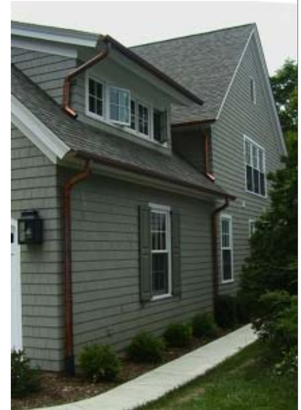
side elevation above the garage
