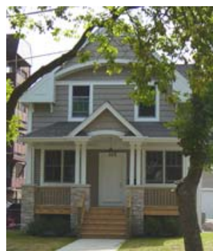
b. 2002, 2 story, frame & masonry construction
