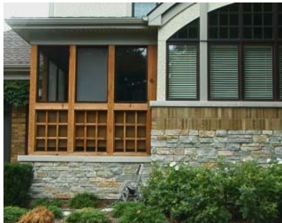
new addition: a well balanced new facade and elevation
