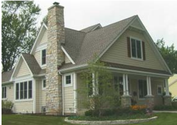
side elevation with a projecting bay
