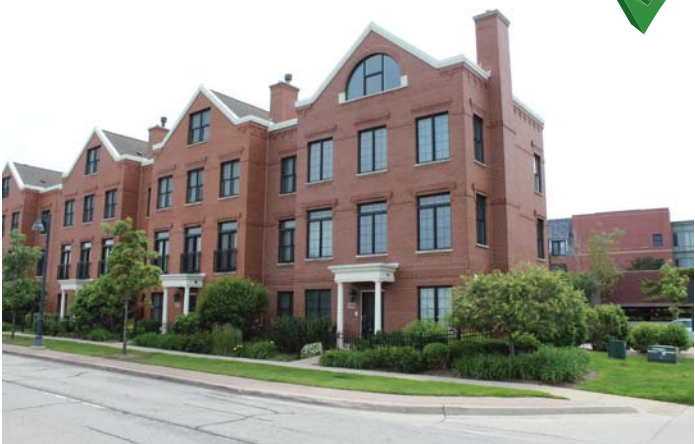
Front building facade facing major road
