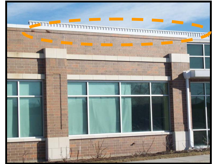
An appropriately designed screen hides roof-top mechanical units from the view of the parking lot and the public right-of-way.
