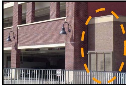
(2). Equipment is shielded from the right-of-way with a masonry structure attached to a parking garage.
