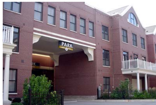
The parking deck is effectively screened by a building (6)
