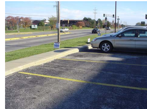
No perimeter landscaping is provided to screen cars from the public view(1)
