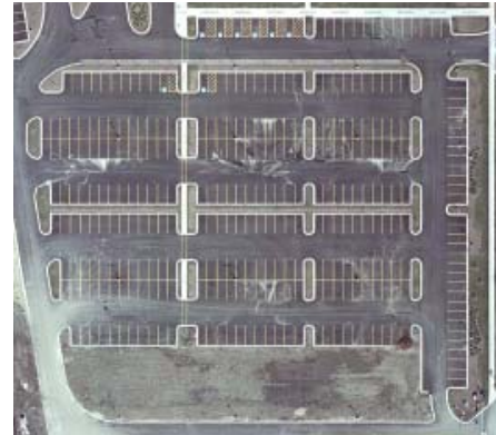
A large parking area is divided into smaller parking fields with large landscaped islands (3)
