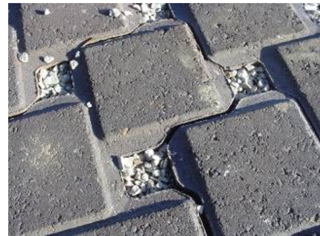
Porous parking lot materials incorporated as part of the overall parking lot plan allow storm water to be absorbed gradually (4)
