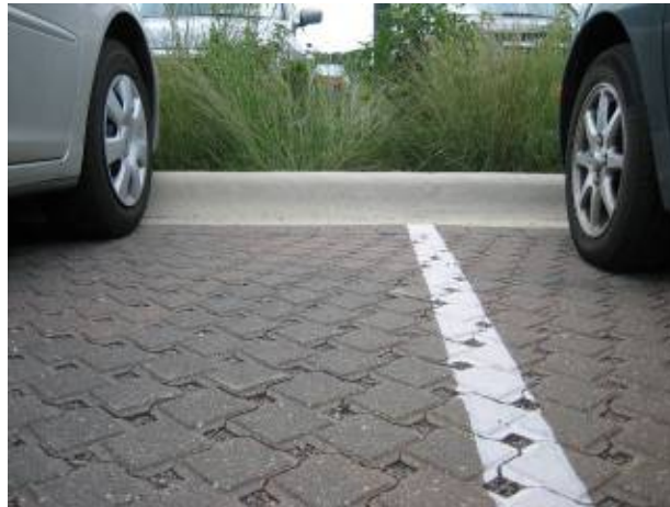
Porous parking lot materials incorporated as part of the overall parking lot plan allow storm water to be absorbed gradually (4)
