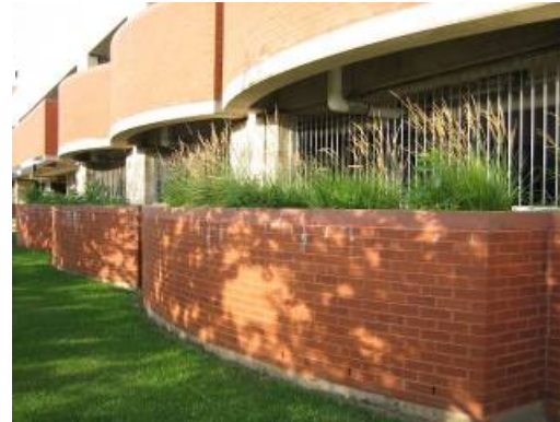
Planting boxes or climbing vines can be used around the exterior of the parking deck (4)
