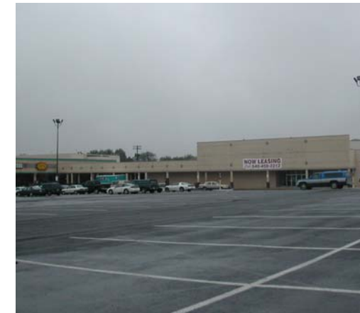
A large parking area that has no landscaping islands or trees (1) (Courtesy of the Coalition for Smart Growth)
