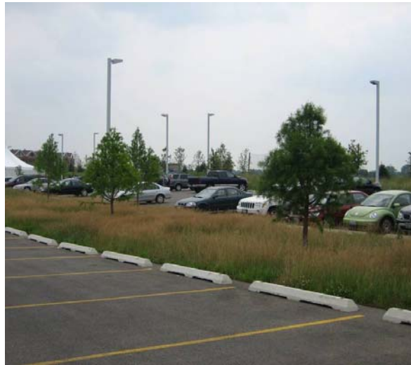
Bioswales incorporate native wetland plantings for stormwater drainage(1, 3)
