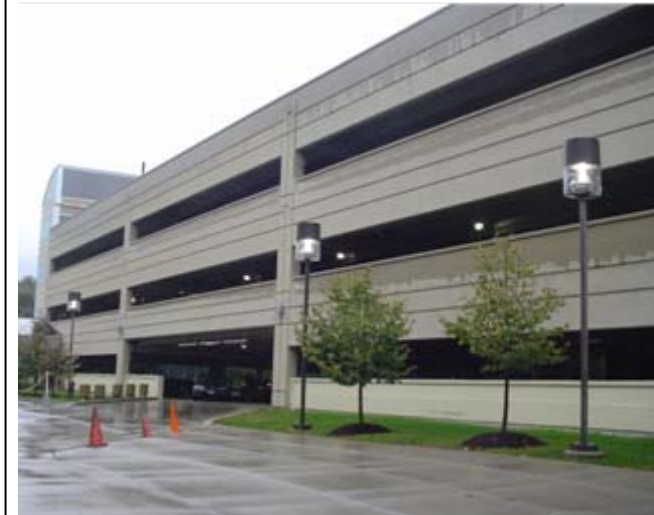
Planting boxes, trellises, or hanging boxes should be used to enhance the exterior of the parking deck (3)
