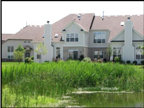
Naturally landscaped detention pond consisting mainly of grasses and reeds.
