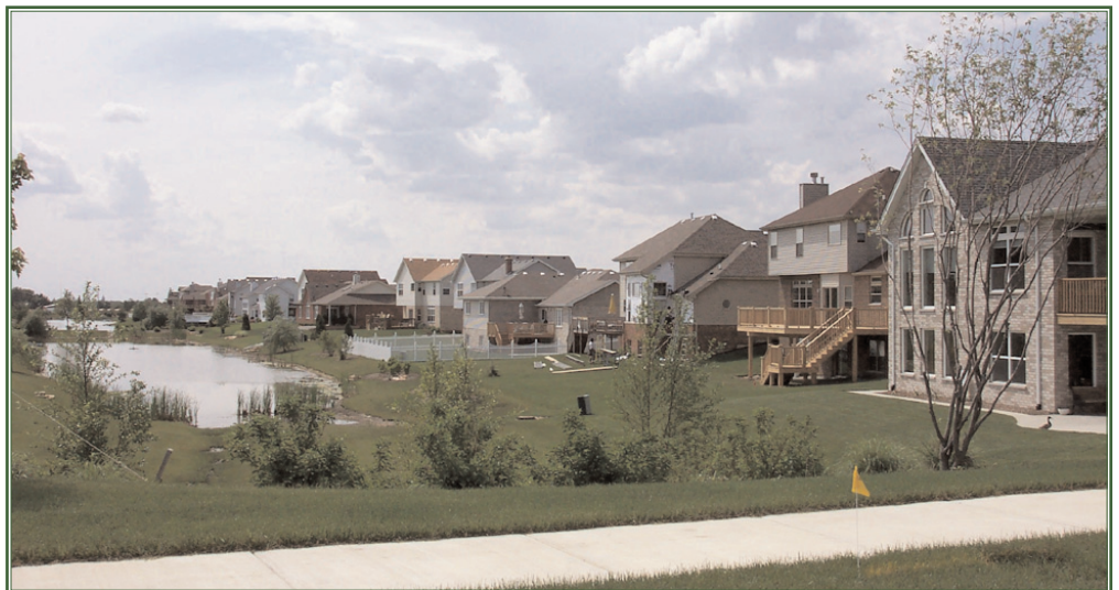
WATER RETENTION POND
