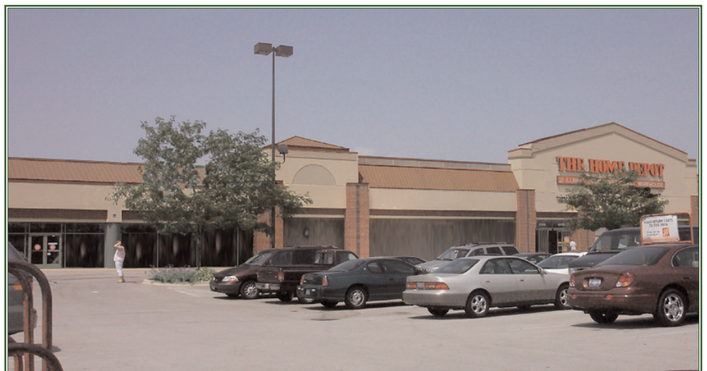
A COMMERCIAL BUILDING WITH GOOD SIGNAGE, COLOR AND NO OUTSIDE DISPLAYS
