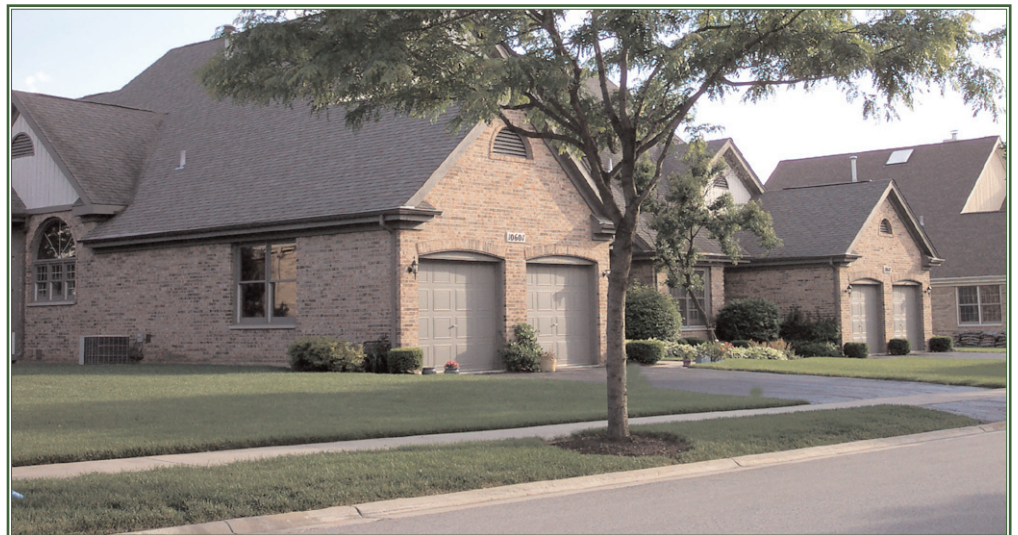
TOWNHOME GARAGE DOORS - BEFORE
