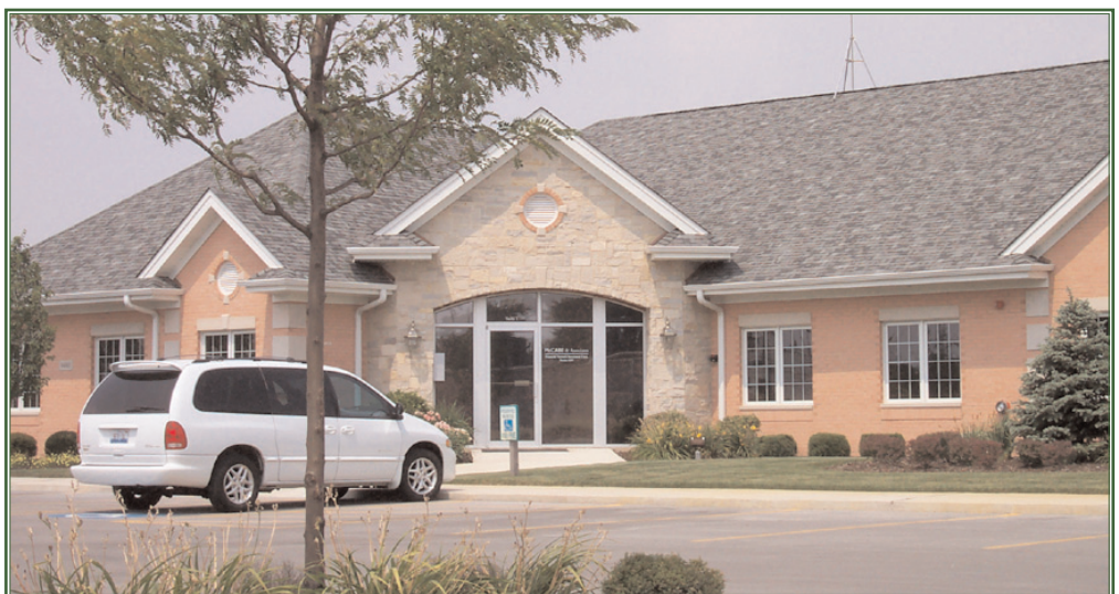
COMMERCIAL BUILDING WITH GOOD MATERIALS AND COLOR
