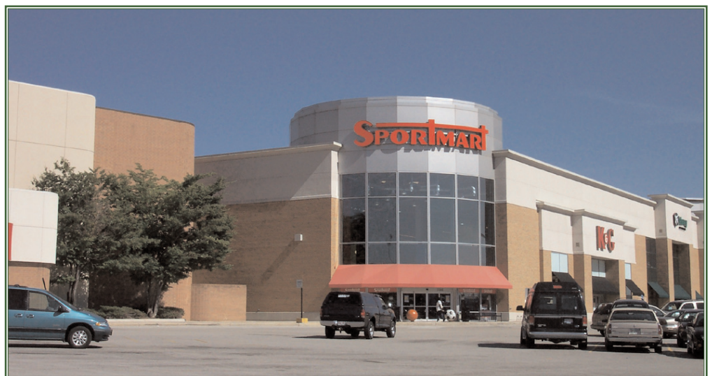
A GOOD EXAMPLE OF A COMMERCIAL FACADE
