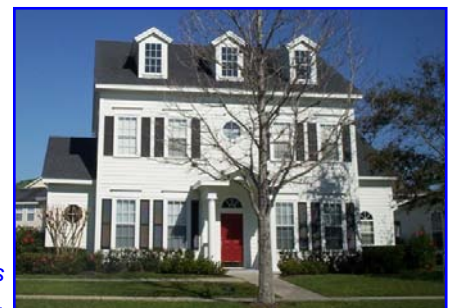
Example of shutters on front elevation.
