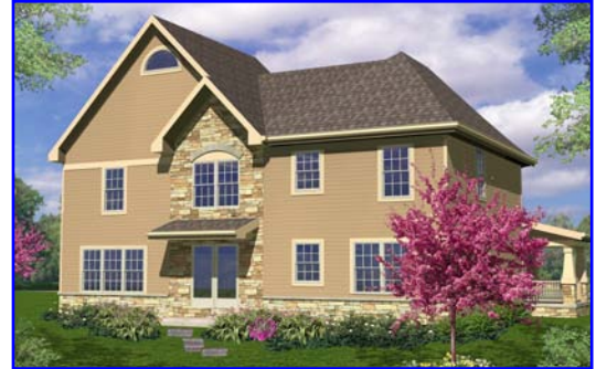
Example of balanced windows on rear elevation.
