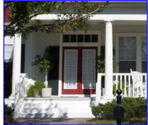
Good use of door transom.
