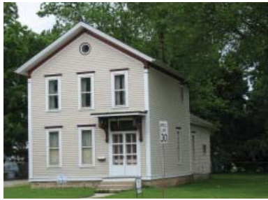
Top: I-House close to the expanded downtown with a side gabled roof, three bays, and gabled front entry with paired columns.
