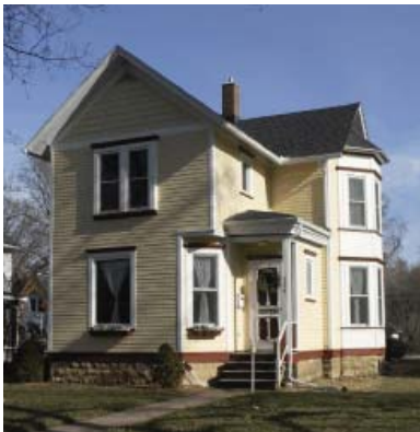
Above: Side Hall Plan residence with Italianate influences, including a gabled roof, corner boards with plaster caps, and flat roof door hood with brackets.
