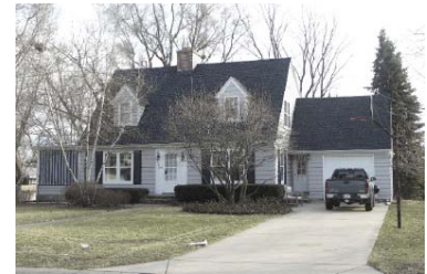
Top: A Colonial Revival on Center Street with a bay window, dormer window, symmetrical facade and Doric porch columns.
