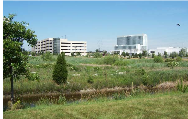
Old Unocal Detention Basin (west of Ikea)
