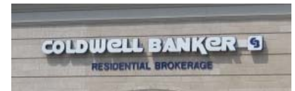
Raceway does not extend beyond sign face.
