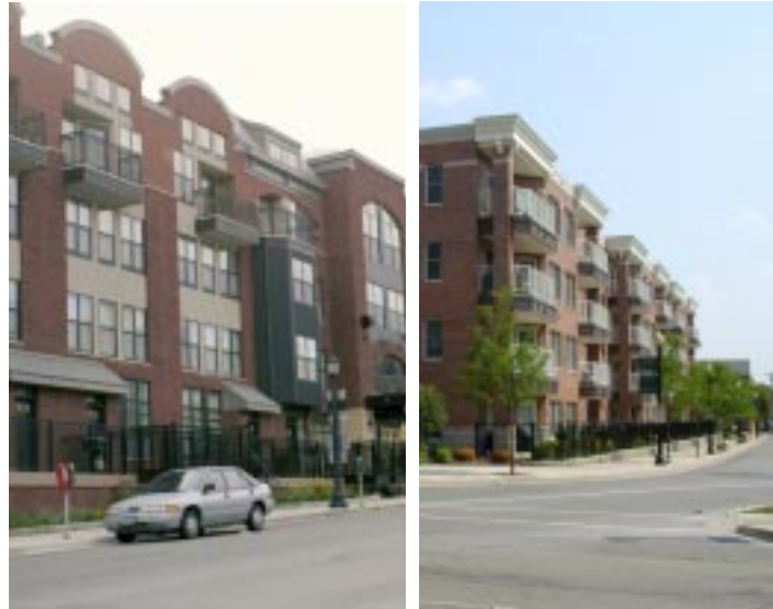
Buildings that lend a sense of activity to the street with usable balconies are highly encouraged
