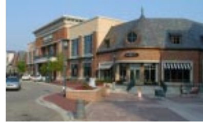
The use of quality materials, ones that lend an enduring quality to new buildings, with scales and forms that feel right to pedestrians are the goal for First Street
