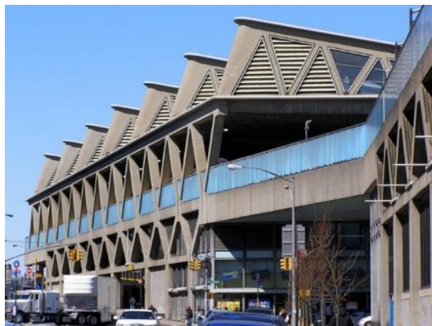
The refurbished George Washington Bridge Station at 179 th Street in northern Manhattan. This station’s bus pavilion on the third level became a focal point for Greyhound’s Northeast Corridor expansion in 2017. (Flickr photo)
