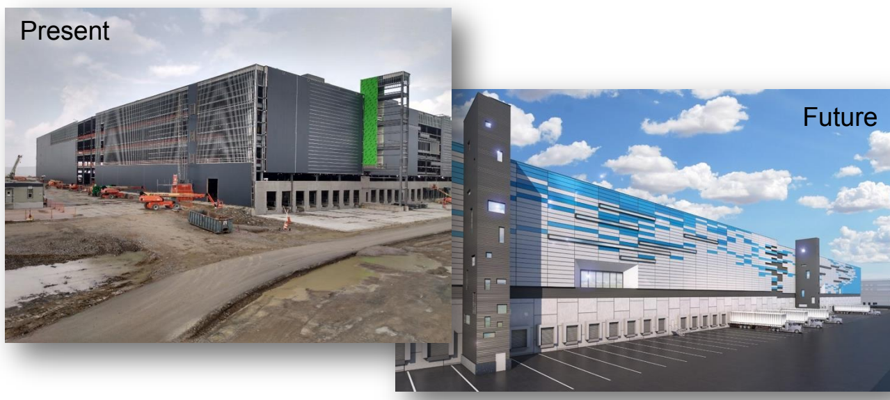
Amazon’s massive complex at Cincinnati CVG, pictured above on August 5, 2020, is in the final stage of construction. The airside portion of the structure is in the distance. Pictured at right is an Amazon-commissioned drawing of how the structure will look and how the truck bays will be used upon completion (left, Chaddick collection; right, Amazon).
