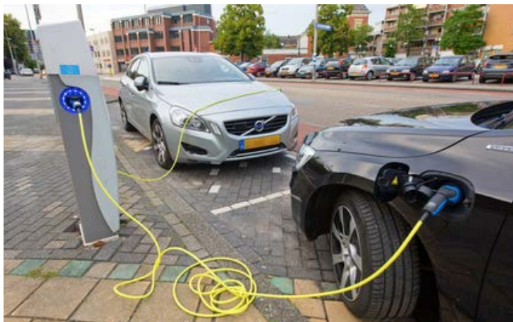
An electric car charging station in the Netherlands.
