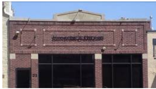
Pin-mounted letterforms should contrast with the background material, not blend in so that the sign is illegible (2c)
