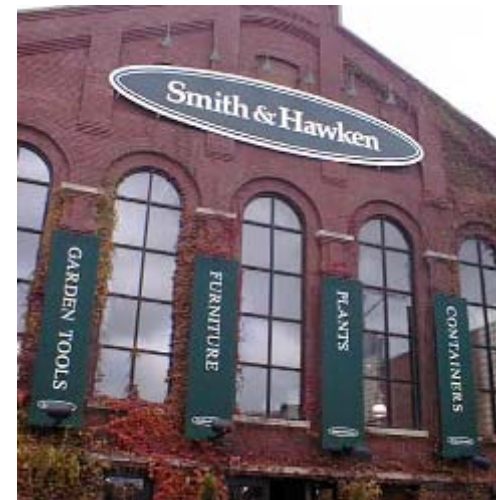
Wall signs are preferred to be placed no higher than the first floor (1c4)
