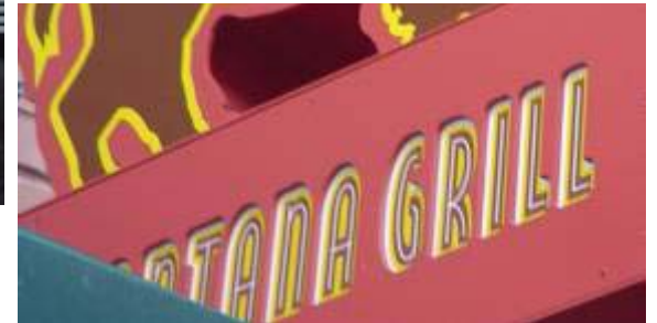
A blade sign is routed out and uses back-up acrylic forms.
