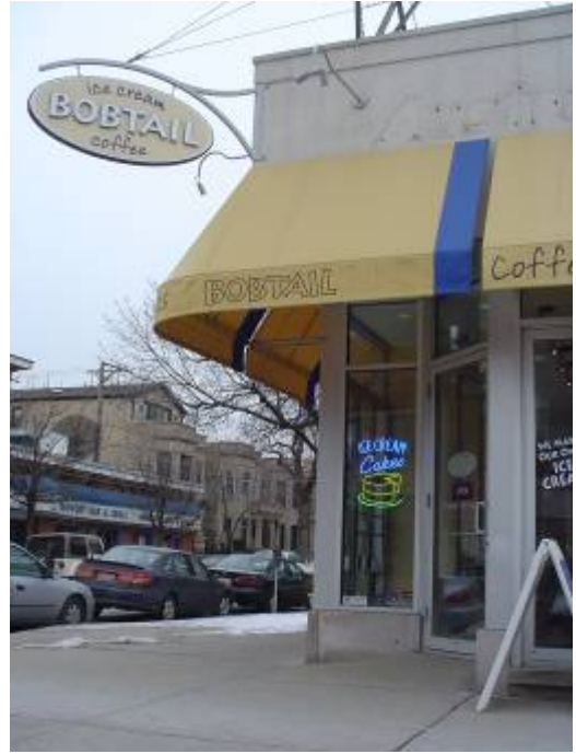
Blade sign is attached with wiring from the roof and is oriented toward automobile traffic (4a1)
