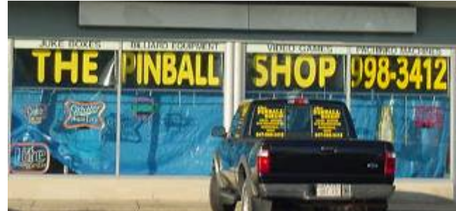
Low-quality materials completely obscure visibility into the storefront (3b, 3e)
