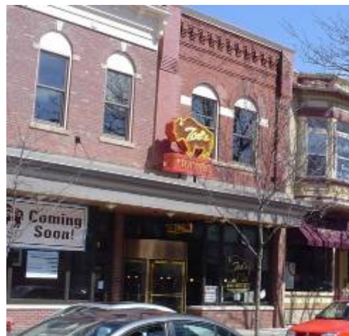
A well-designed sign is located inappropriately on the building (1c2)
