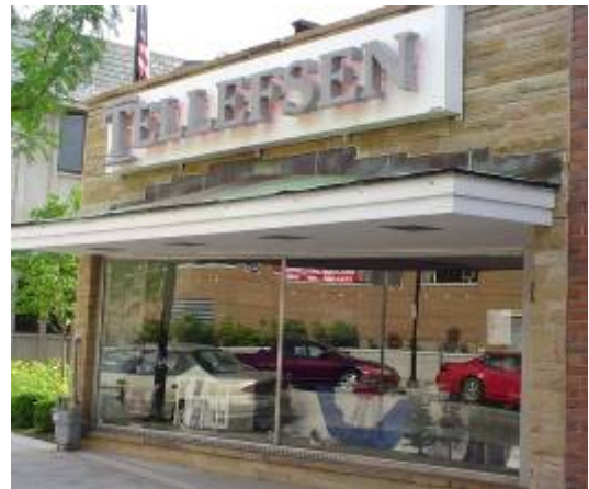
Pin-mounted letters on an obtrusive box that projects from the storefront (2b)
