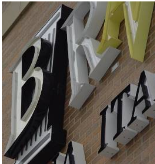
Wall sign illustrates exposed neon in metal channel letterform with a matte acrylic face (1d2)
