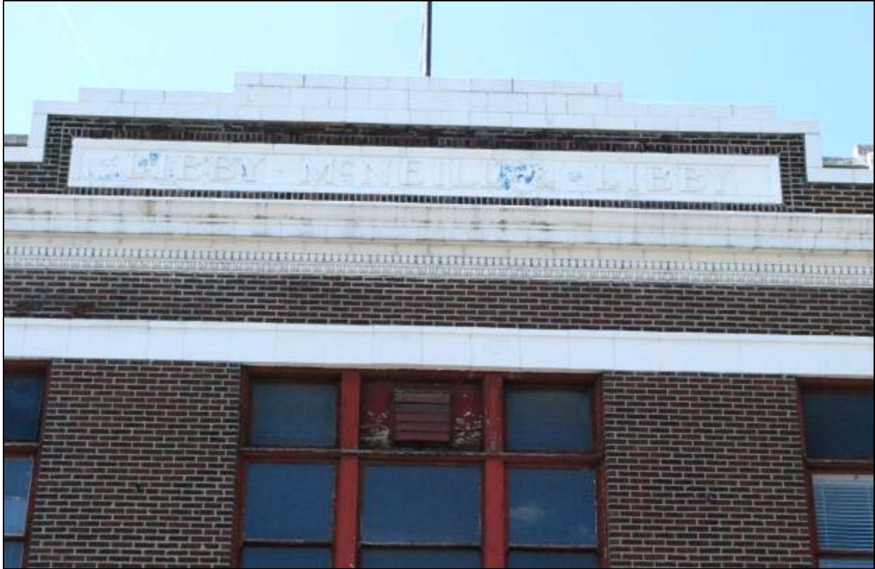
Image 12: Parapet detail of Office Building with “Libby McNeil & Libby” terra cotta panel (2012)
