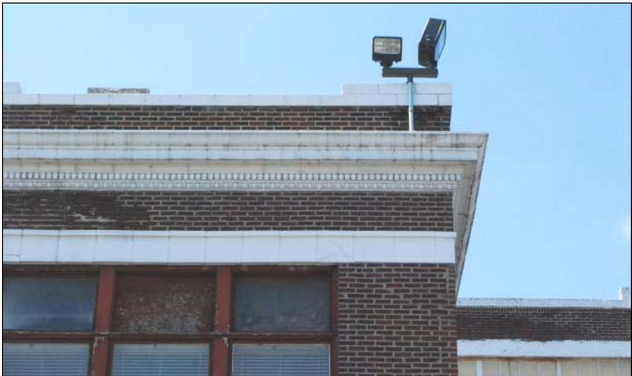
Image 13: Terra cotta cornice detail on Office Building (2012)
