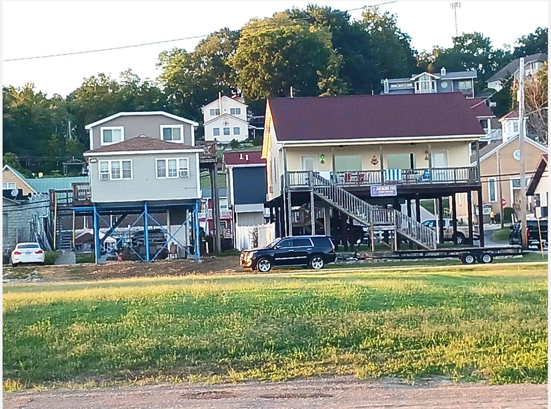
Housing in Grafton elevated to reduce damage from periodic Mississippi River flooding.
